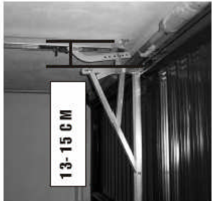
Fix the lever of the trolley to the telescopic arm using the 3 rd or 4 th hole of the lever.
